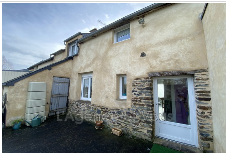
House La Fresnais
